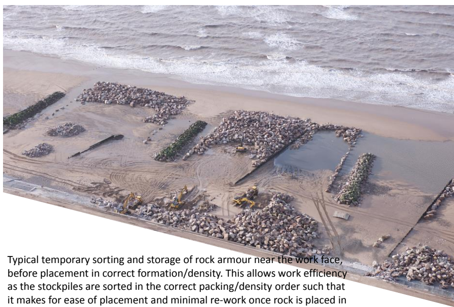
Figure 10- Typical rock armour storage near work face
