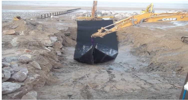
Figure 18- Typical geotextile placement
